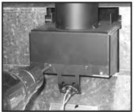
Figure 35: Install Spill Switch on Bracket.
